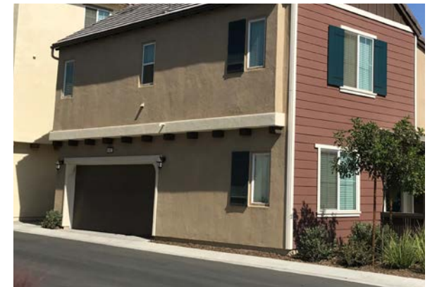
Unsuccessful Drive-aisle treatment in limited space
