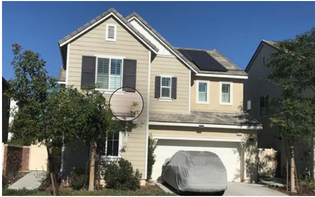
Horizontal Siding at primary exposed area
