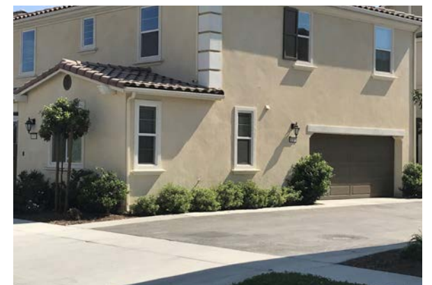
Successful Drive-aisle treatment in limited space
