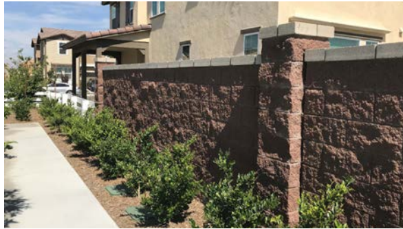
16" Square Column at exposed side yard and in between homes
