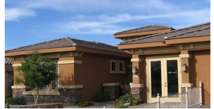
Massive square porch columns with brick or stone base
