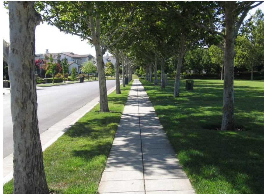
Curb Separated Sidewalks
