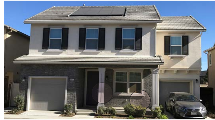
Stone or brick veneer accents Simple wood columns and railings at porch
