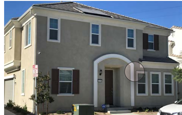
Prominent entry door trim detail
