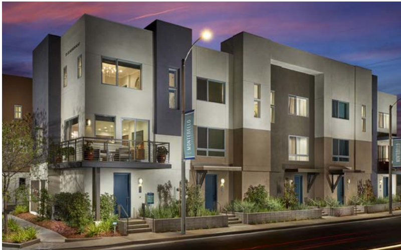
Variation in parapet height, design, and materials with central common open space
