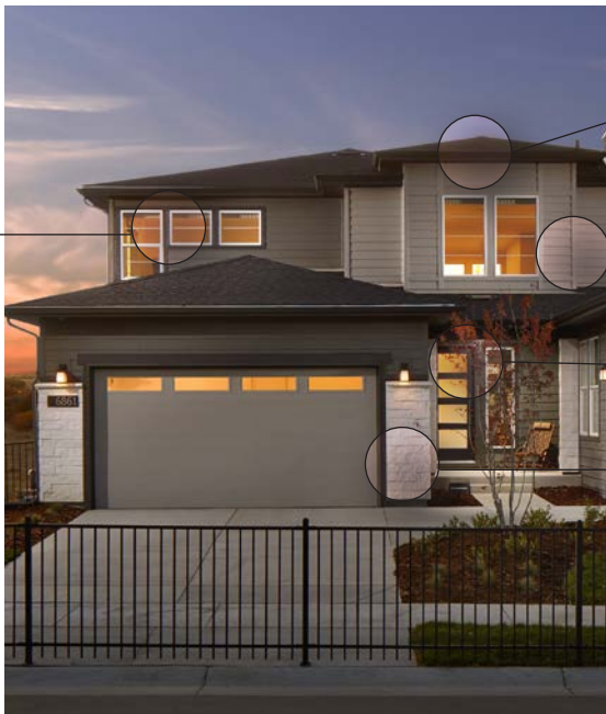
Ribbon windows, generally in groupings of three
