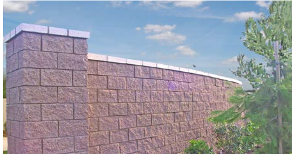
24" Columns along Perimeters
