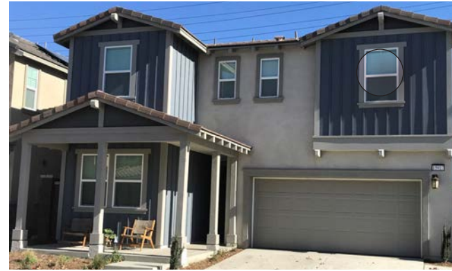
Single-hung windows at front elevation
