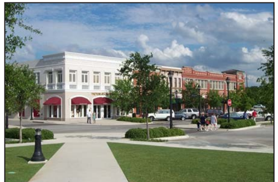
An example of a mixture of retail on the bottom floor and office or residential on the second floor in a Community Core.
