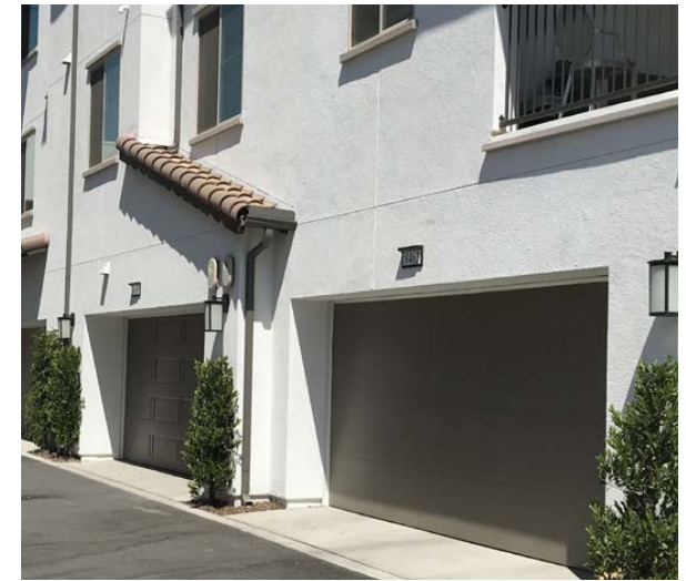
Typical Drive Aisle Condition
